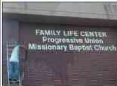
Gullatte Construction at work
