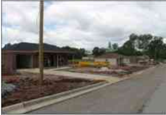
The new Habitat for Humanity community in Northeast Huntsville.
