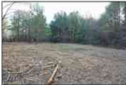
Land being cleared, Jan. 15, 2021
